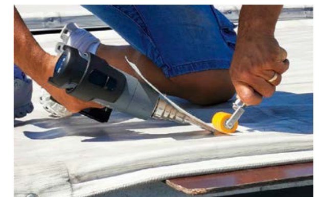
Tarpaulin Roofing Sheets
